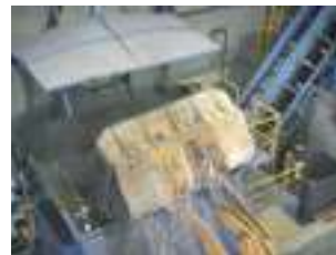
(3) The opening of shredding machine (exclusive access)
