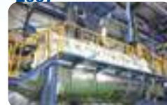
Drying facility was completed
