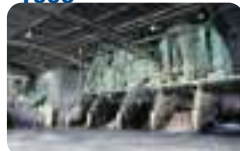
Shredding facility was expanded
