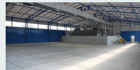
Reverse Management Center (RMC): A dedicated storage facility for waste beverages
