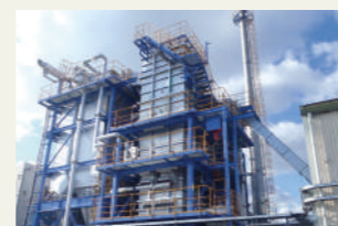
2014 New biomass boiler is installed.
